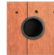
Pipe Pocket in Floor
